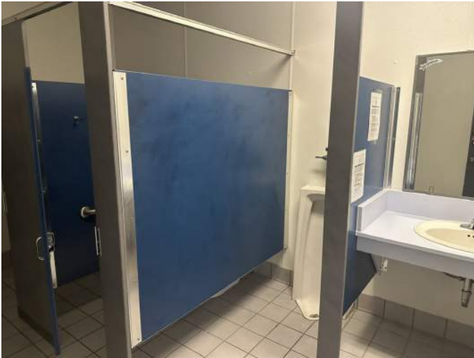
m. Image of Men's Restroom. Note the piping at the Lavatory is missing the protective insulation.
