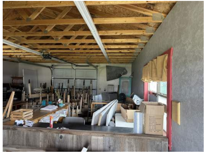
d. Image depicts the interior of the building looking South.
