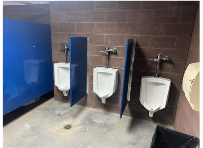
p. Interior Image of Men's Restroom.
