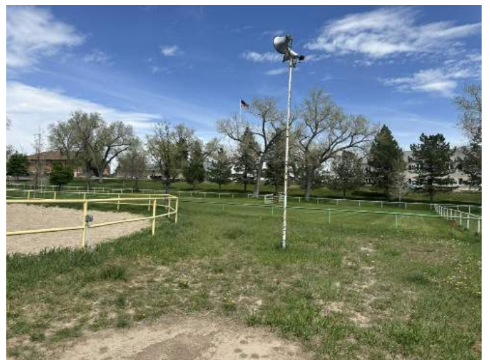
f. Image of the pole mounted speaker system. Note the cable for the PA system wrapped around the pole and running above ground, at grade.
