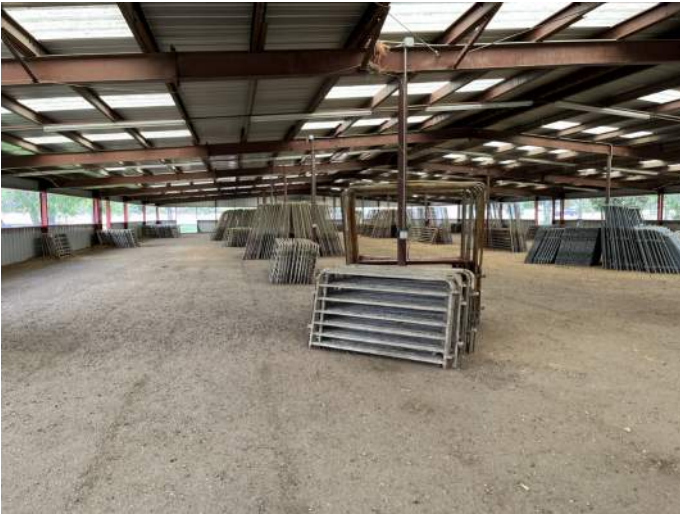
a. Image of the interior of the Sheep Barn looking North.
