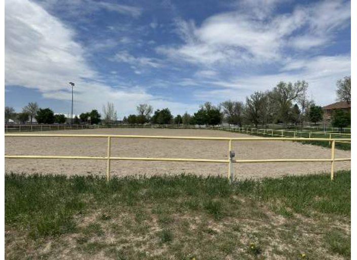
b. Overall image of the Yellow Arena looking North.
