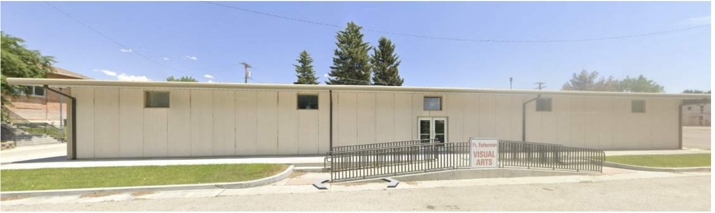
a. Image of the West Facing Elevation
