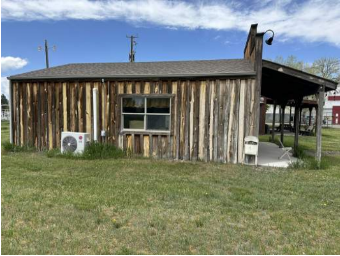
a. Image depicts the East side of the building.
