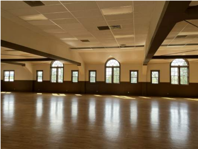
q. Image of the interior of Reno Hall looking West. Note the Rectangular and Palladian Style punched openings.
