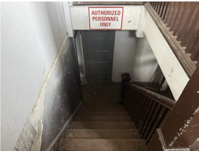
y. Image of Stairs leading to basement.
