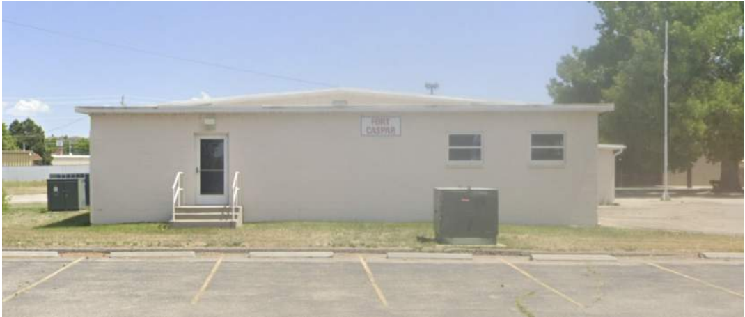
b. Image of the West Facing Elevation.
