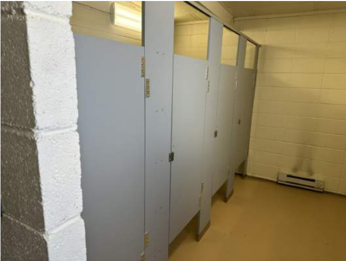
j. Image of the Women's Restroom.
