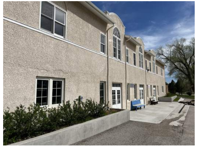
c. Image of West Facing Elevation.
