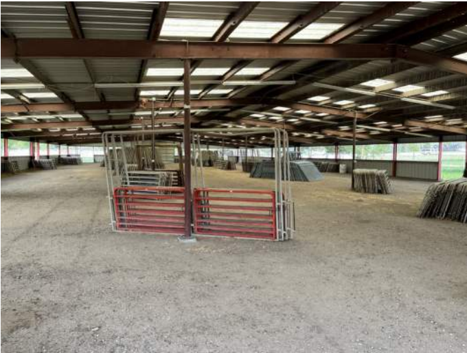
c. Overall image of the interior of the Sheep Barn.
