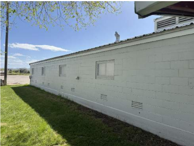
c. Image depicts thru-wall vents and aluminum windows.
