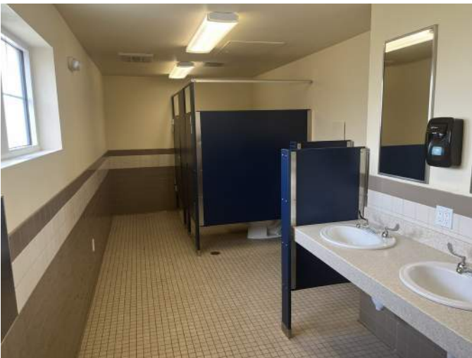
q. Image of the Men's Restroom. Note: The restroom appeared to be wheel chair accessible.
