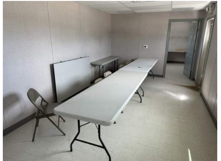
d. Image of the main meeting space at the Rodeo Office. Note the dirt that appears to have blown in under the door. Inspect the seals and sweep where the bottom of the door and sill meet and replace if needed.
