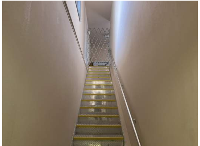
f. Image of the interior stair leading from the Ground Floor Level to the Upper Level, Reno Hall.
