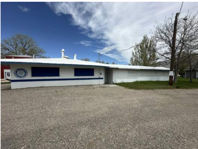
e. Image of Southeast facing facade with the Dining Pavilion visible in the right side of the image.
