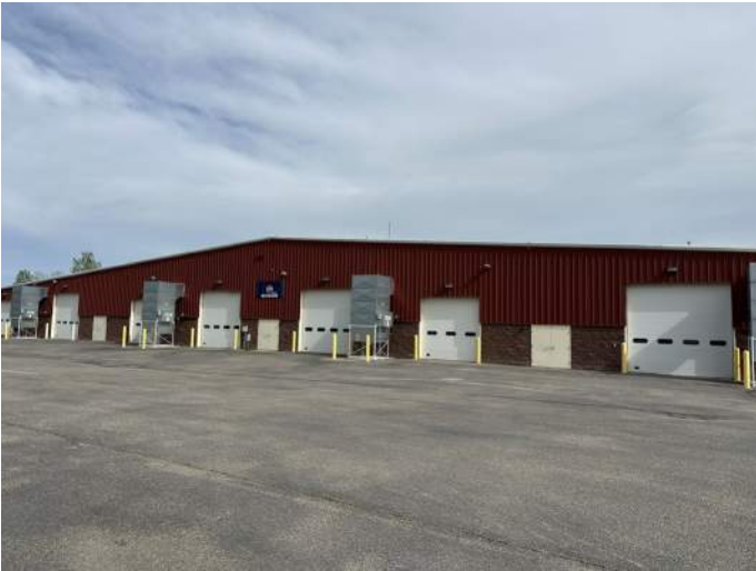
c. Image of South Elevation of the building.
