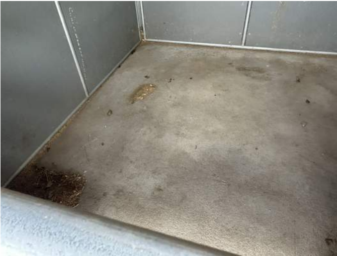
i. Image of typical interior of equine stall floor for Stall Barns 'A' and 'B'.
