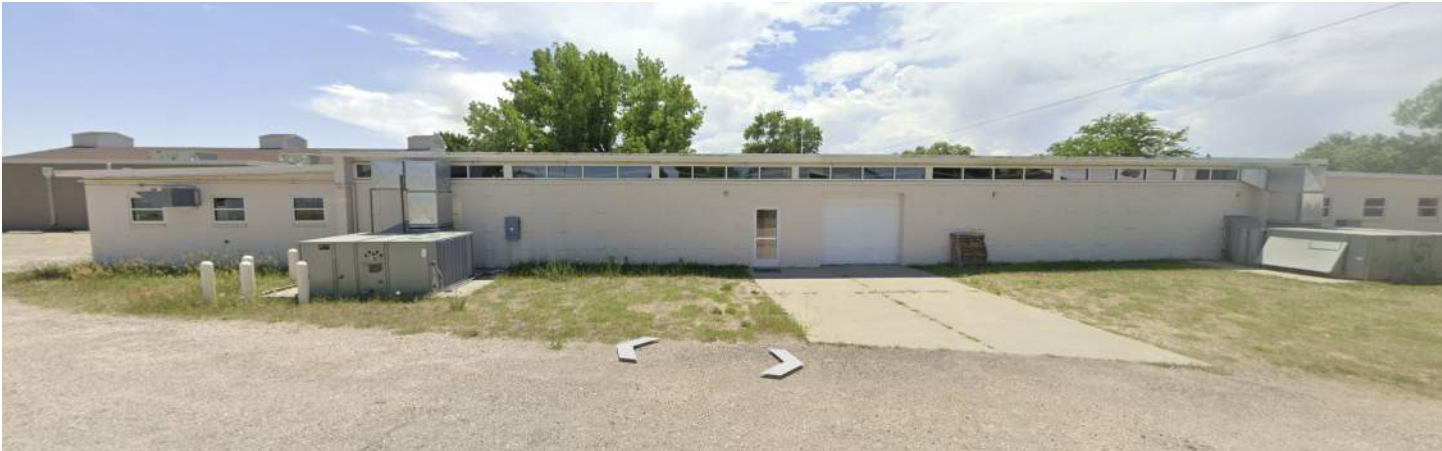
c. Image of the North Facing Elevation.
