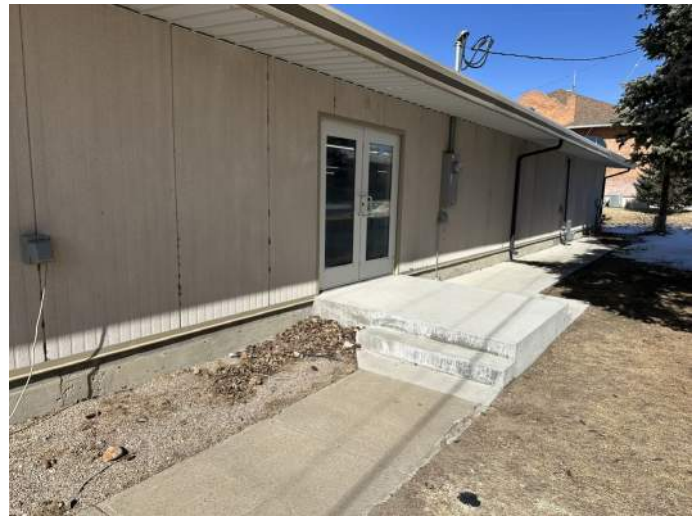
c. Image of the East Facing Elevation.
