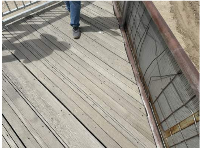
b. Image of the existing observation deck and landing.
