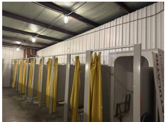
f. Image of shower stalls.
