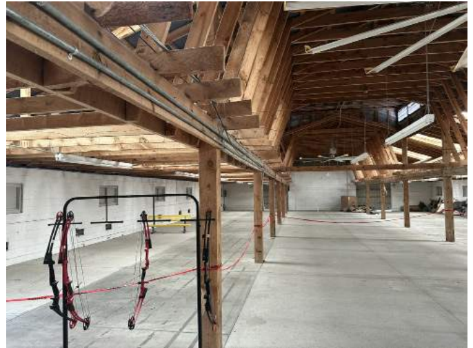
n. Image depicts roof structural system.
