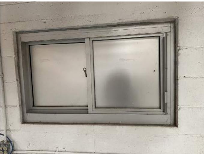
e. Image depicts an existing aluminum window with infill panels.
