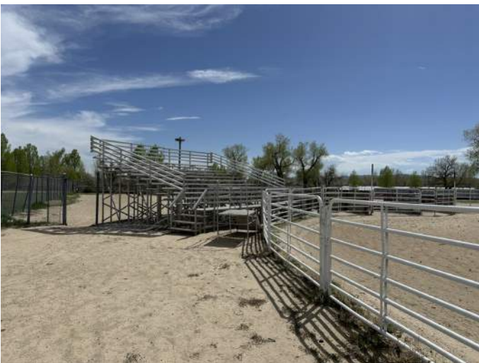
e. image depicts aluminum bleachers located by roping chutes. Note, the bleachers are not ADA accessible.
