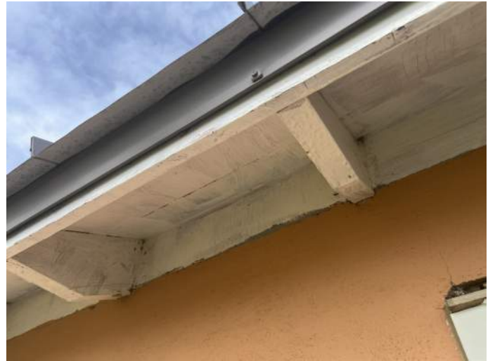
j. Image of paint application on beams and soffit.
