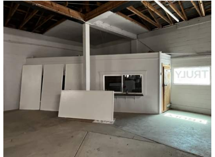
b. Image depicts existing walk-in cooler converted into an office.
