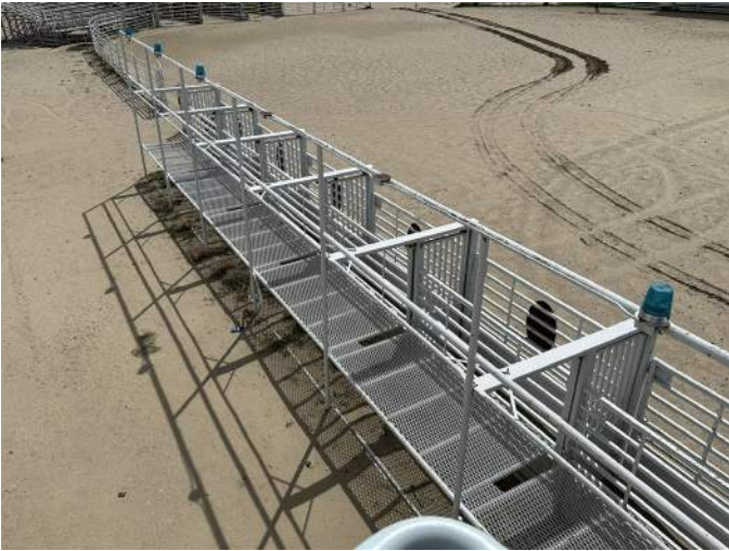
g. Slider gates at the stock chutes require maintenance and or replacement as they are difficult to operate; and can effect the flow of competition events.
