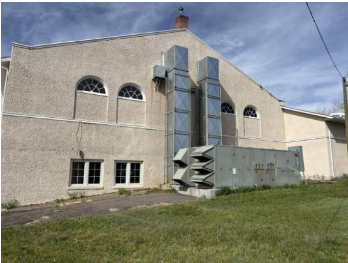
b. Image of South Facing Elevation. Note the packaged air units.
