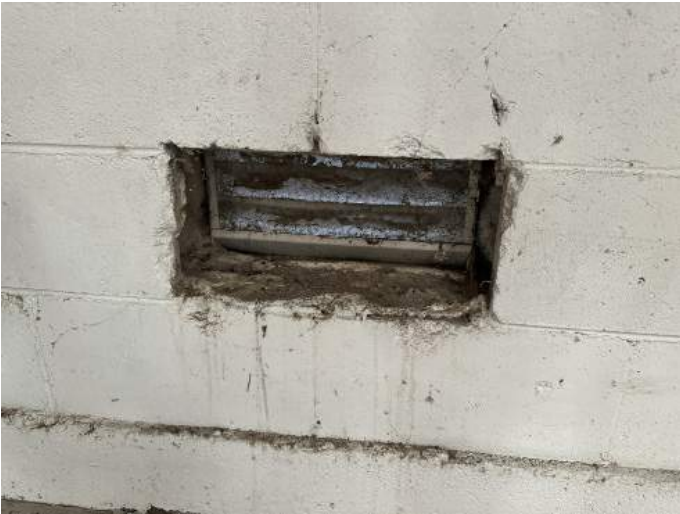
a. Image depicts existing thru-wall vents.
