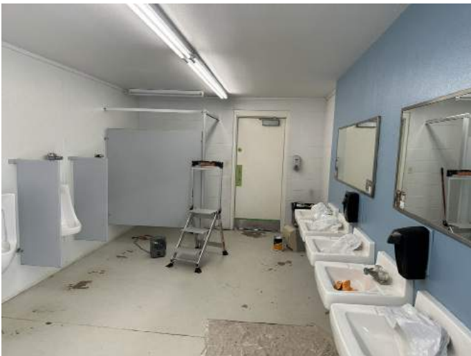
e. Image of the interior of the interior of the Men's Restroom. Note the height of the mirrors, and missing toilet accessories and faucets with handles that require twisting and grasping.
