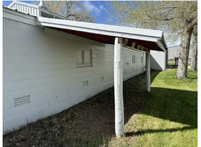
b. Image depicts thru-wall vents and the existing lean-to structure.
