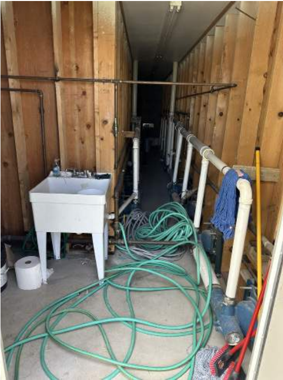
f. Image of the plumbing chase between the restrooms.
