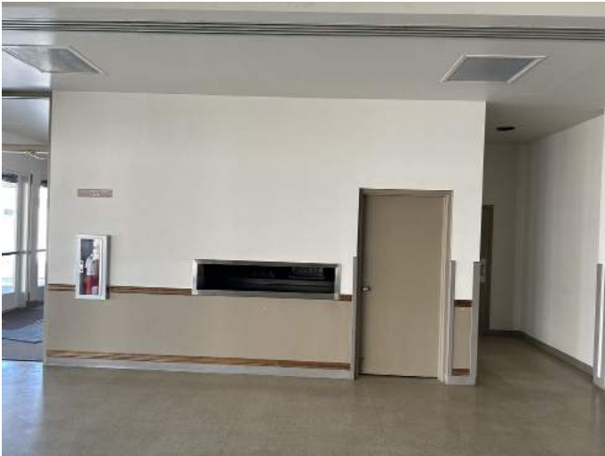
c. Image of the dish return in the multi-purpose space.
