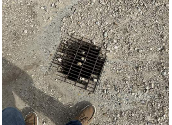
h. Image of existing storm drain. See narrative section titled 'Other.'
