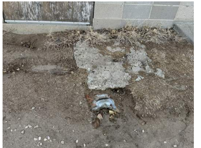
f. Image of a plugged storm drain outlet. Also note the uneven surface in front of the door. c. Image of pre-engineered wood truss and individual equine stalls. The Red Arrow identifies the exposed conductor noted in the narrative.
