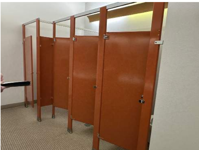
q. Image of the interior of the Women's Restroom.
