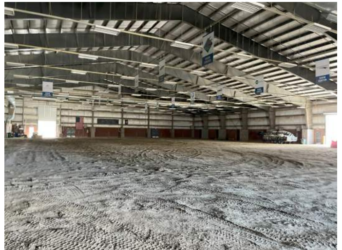
d. Image of the dirt floor within the Touchstone Show Center.
