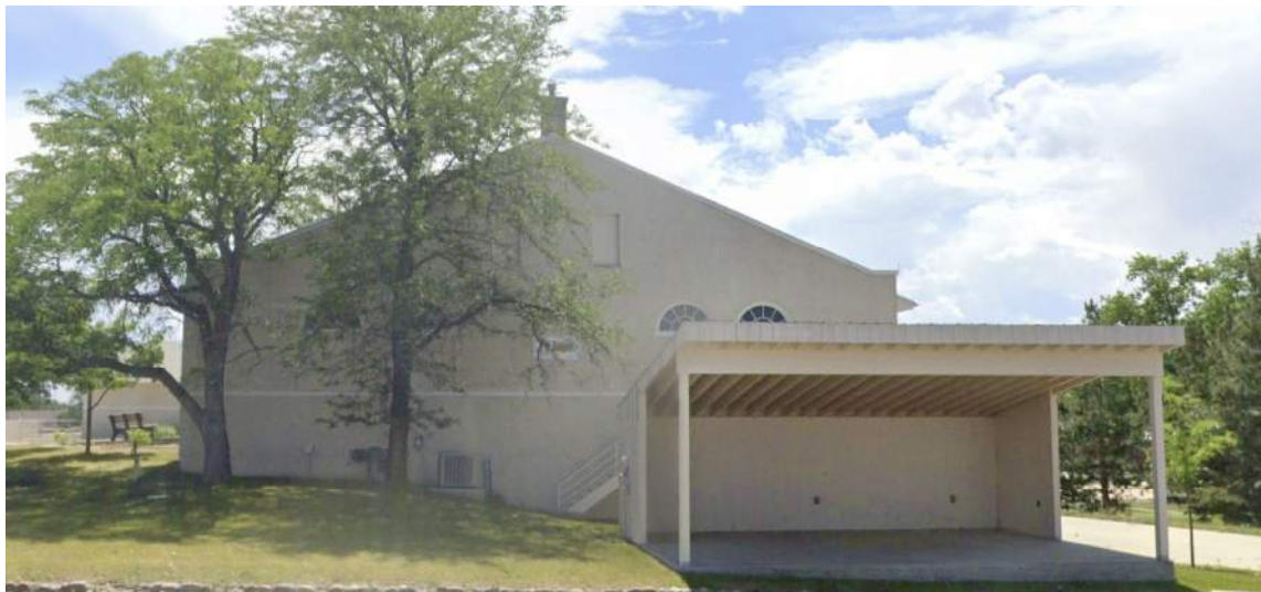
d. Image of North Facing Elevation.
