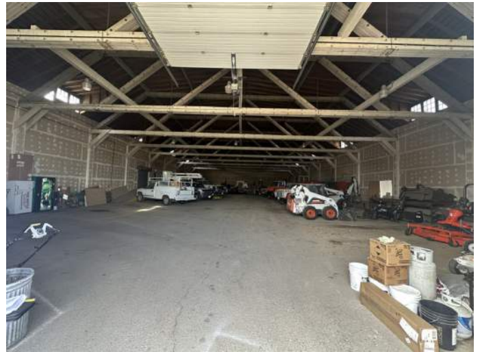
t. Interior Image of Vehicle and Equipment Storage looking North.
