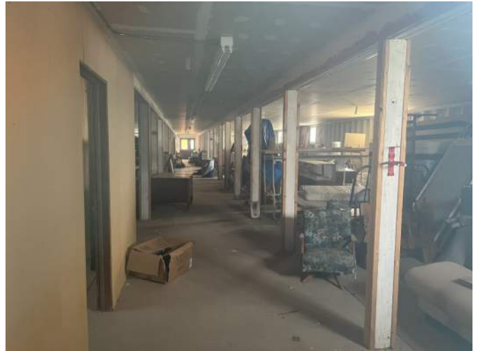
v. Interior image of the ground floor level of the building.
