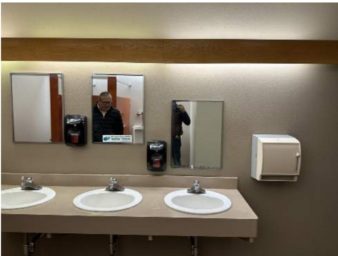
u. Image of the lavatories in the Men's Restroom.
