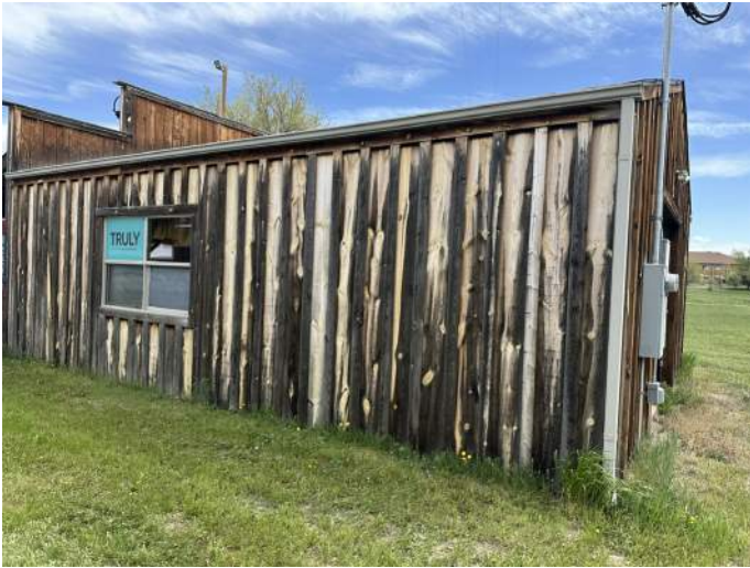
c. Image depicts the West side of the building.
