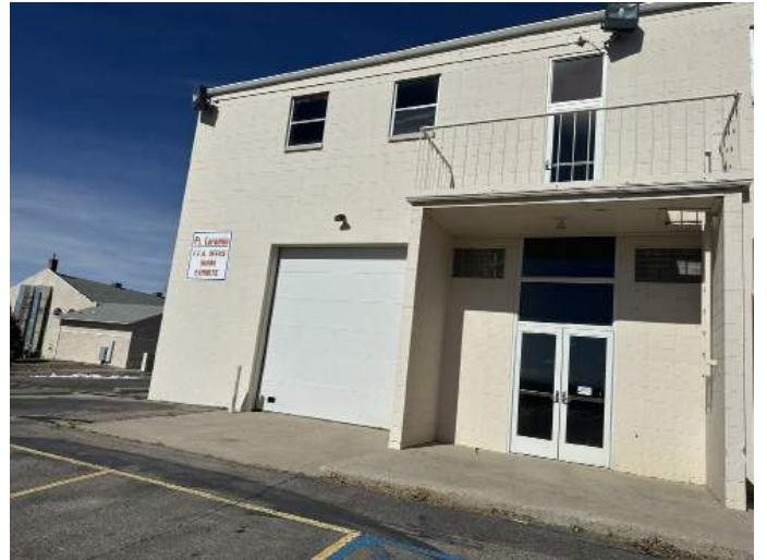
b. Image of the South Facing Exterior Elevation.
