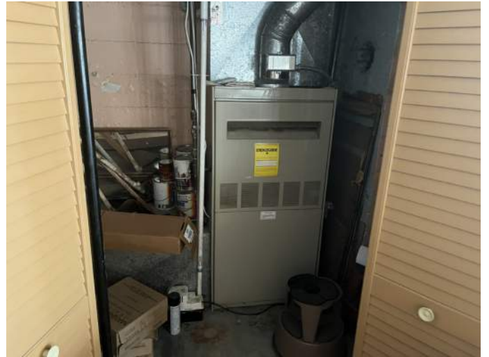
l. Image of the Furnace Closet.
