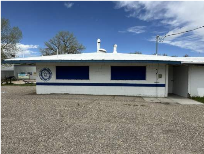
a. Image of the Southeast facing facade of the building.
