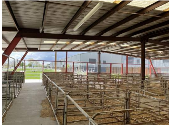
b. Image of the interior of the Goat Barn looking South. Note the electrical panel in the middle of the image.
