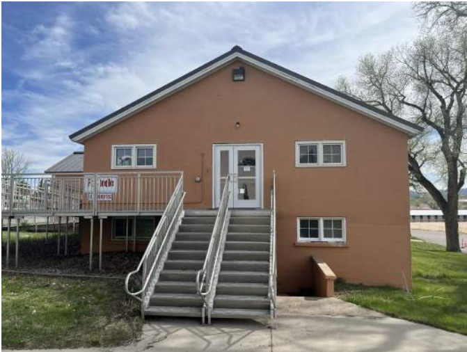
c. Image of the North Elevation facing Fort Reno.
