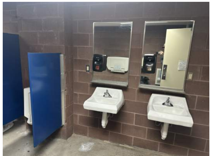
r. Interior Image of Women's Restroom.
