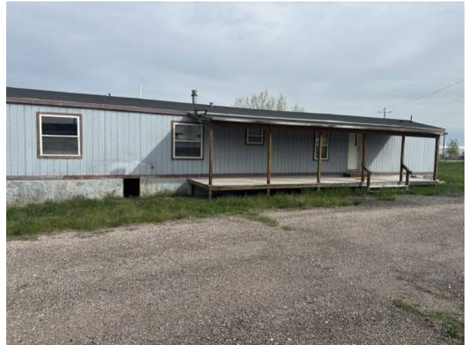
b. Overall image of the exterior of Unit #2.
