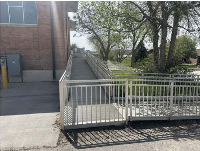
c. Image of the East facing elevation.
