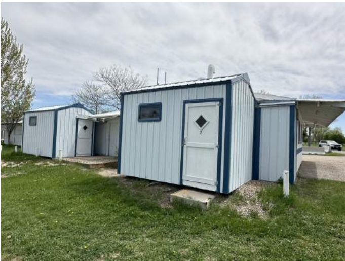
c. Image of the Northwest facing facade with added Storage Sheds.
