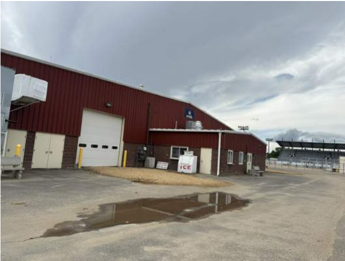
a. Image of North Elevation of the building.
