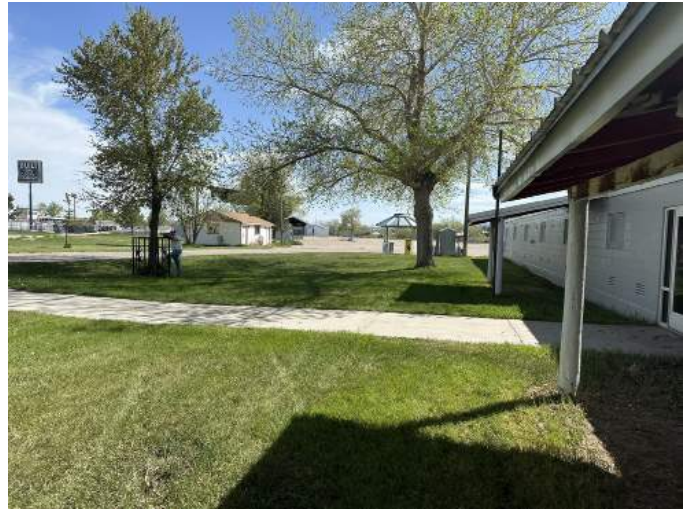
j. Image depicts lean-to's and lawn area at entry to Vyve building.
