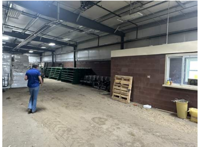
h. Image of Indoor Arena Storage and Support Space.
