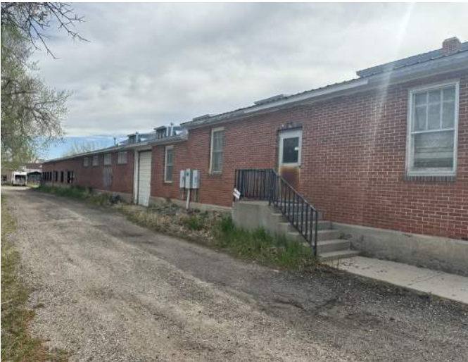
c. Image of the East facing Elevation of the Building. Note the failing paint finish on the metal fascia, improper hand and guard rail at the stair, the exterior hollow metal door that need replaced, stored asphalt paving debris against the building foundation and graffiti.
