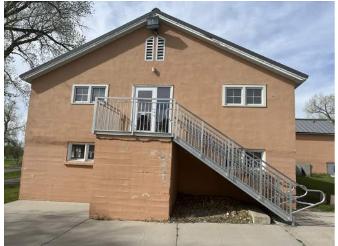
d. Image of the South Elevation facing Paintbrush Lane.
