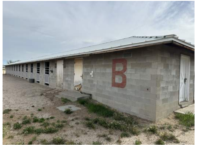
d. Exterior image of Stall Barn 'B'.
