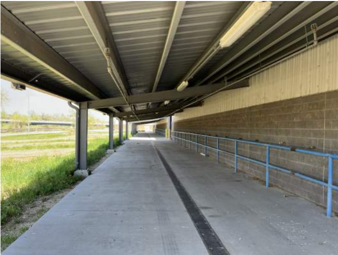
g. Image of Wash Bay with integral trench drain looking North.
