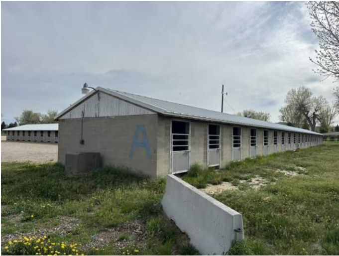
a. Exterior image of Stall Barn 'A'.
