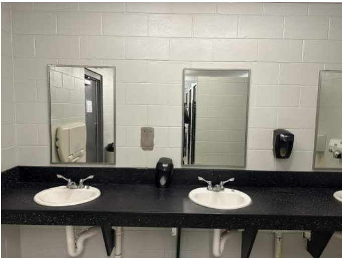
e. Image depicts the soap dispenser that has come off of the wall.
