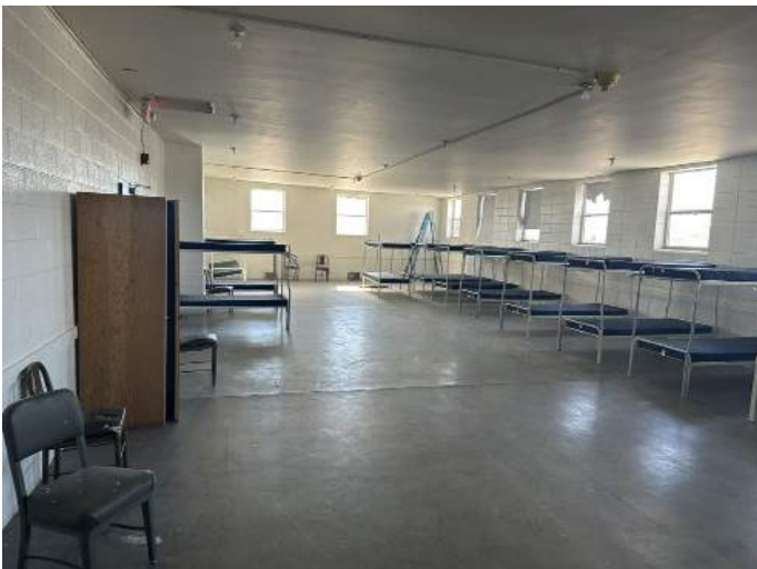
e. Image of a barracks style dorm room.
