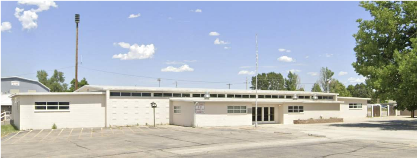
a. Image of the South Facing Elevation
