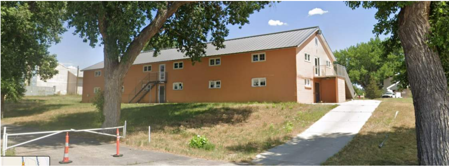
b. Image - West Elevation fronting Paintbrush Lane.
