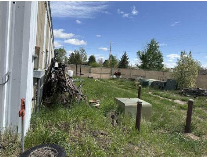
e. Image of debris in the storage building yard along with the transformer and electrical service entry to the building.
