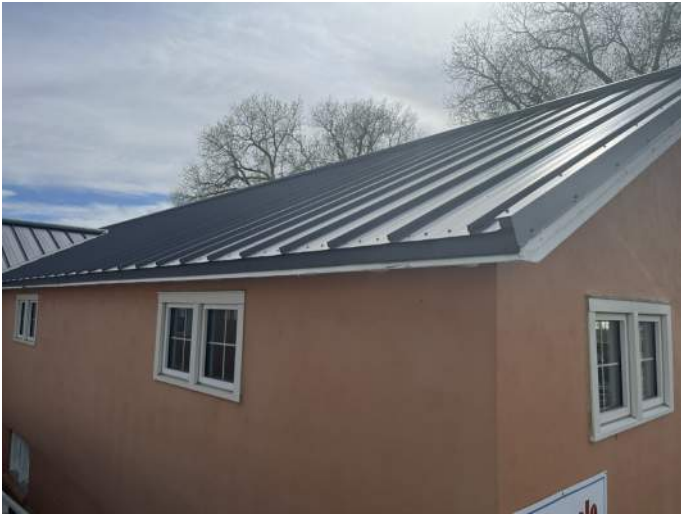
i. Image of paint peeling from the wood fascia. This is a typical condition for all fascia members.
