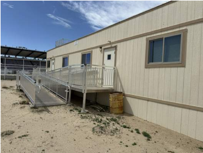
a. Exterior photo of the Rodeo Office + exterior of ADA accessible ramp.
