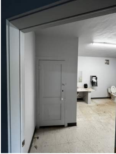
g. Interior of the existing restroom.
