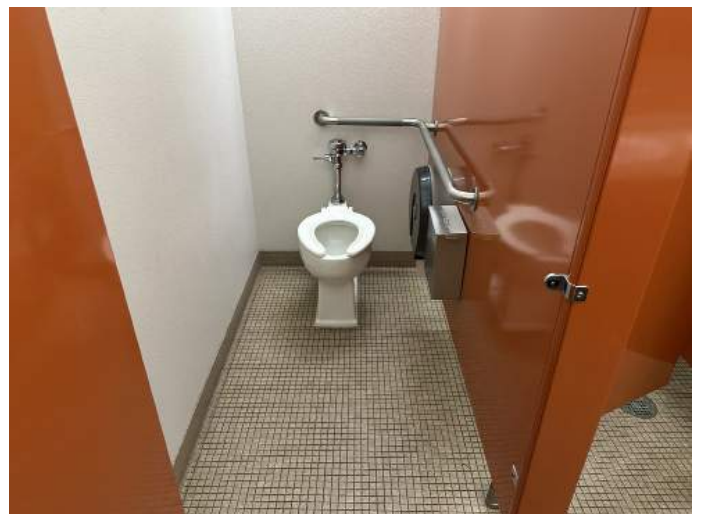
r. Image of a typical toilet compartment within the Women's Restroom.
