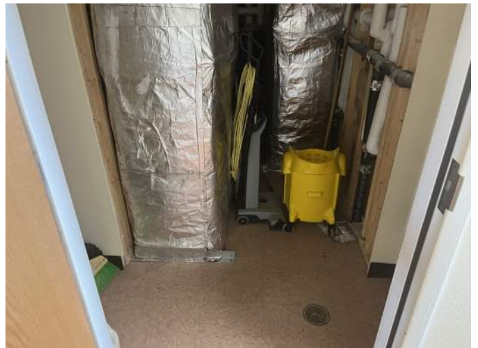
r. Interior image of the Custodian's Closet.
