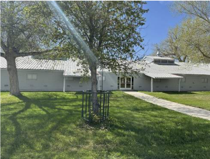
m. Image depicts the East side of the building.
