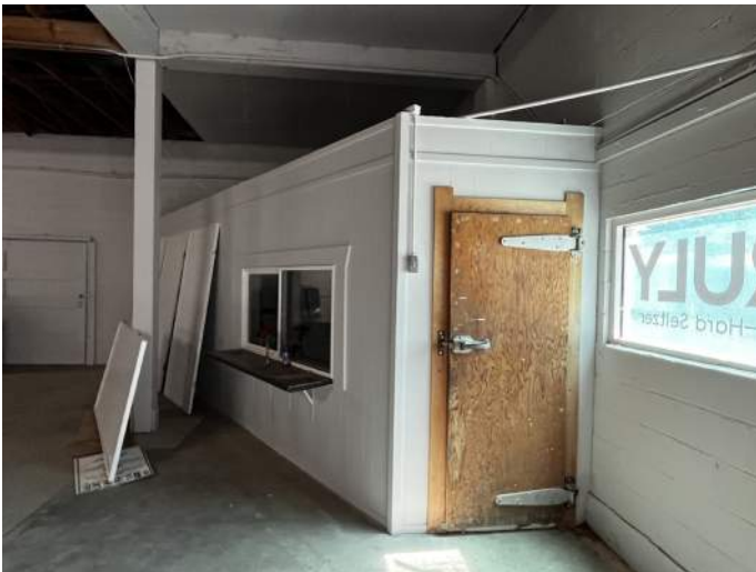
c. Image depicts the original door to the walk-in cooler.
