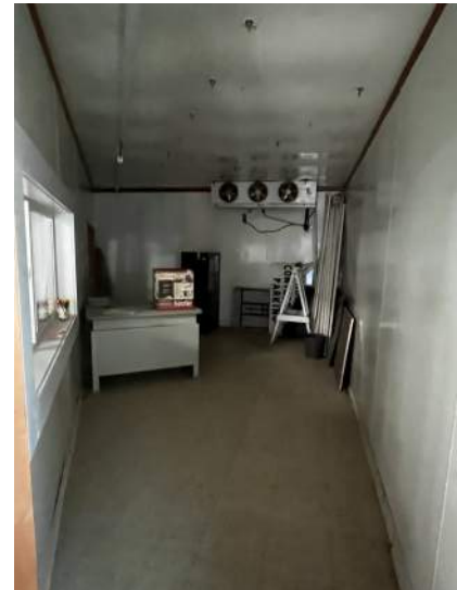
d. Image depicts the interior of the walk-in cooler.
