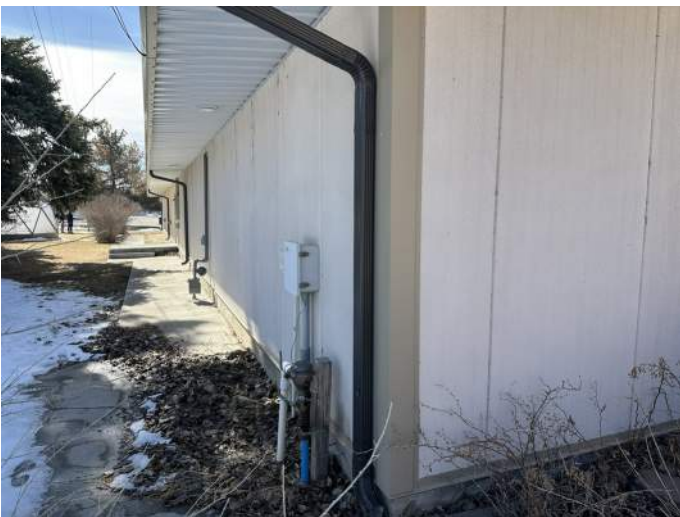
d. Image of the East Facing Elevation. (Additional)
