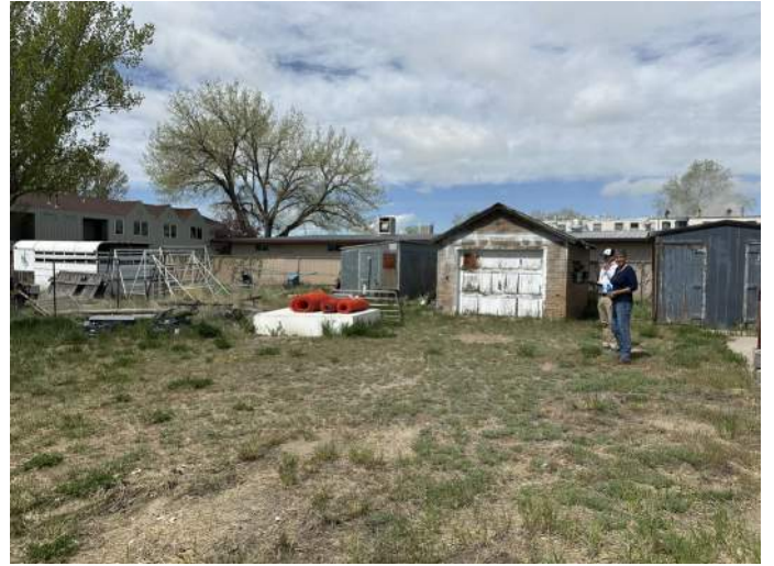
b. Image alternate entry to the Multi-purpose Room. Note the residential patio and front door, improper hand and guard rail, and spalling concrete landing and steps. (North Facing Elevation of the Building.)
