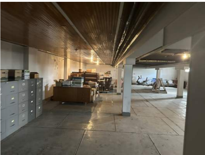
aa. Image of Basement looking West.
