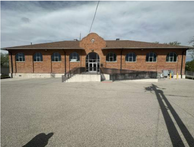
a. Image of the West facing elevation of the building.
