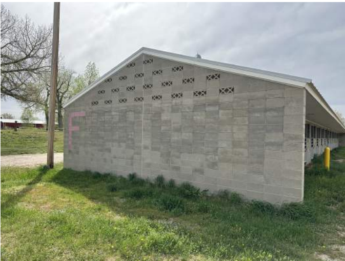
k. Exterior of Stall Barn 'F' as viewed from the North.
